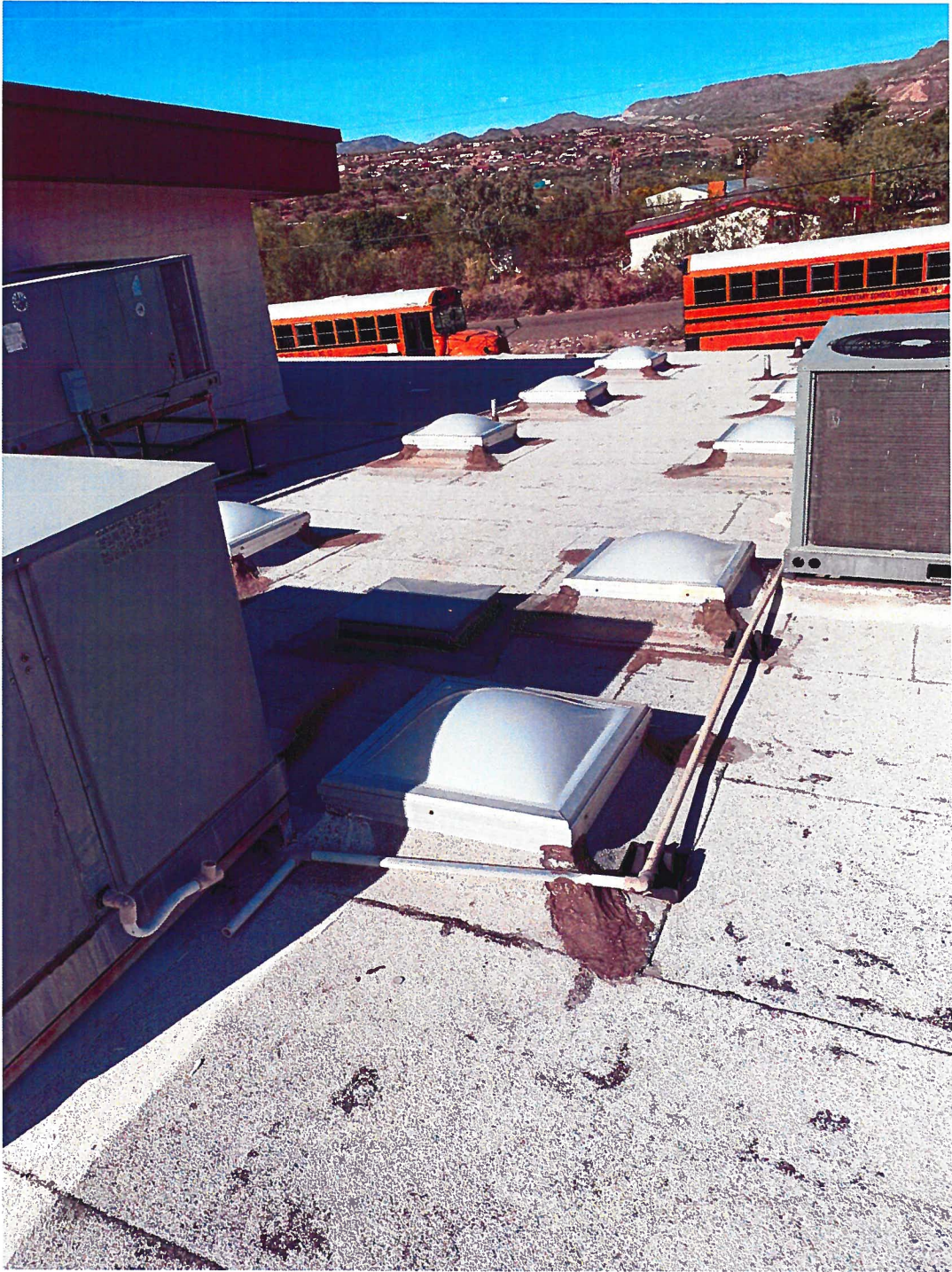
Building 1002 Typical Condition (Lower Roof)
