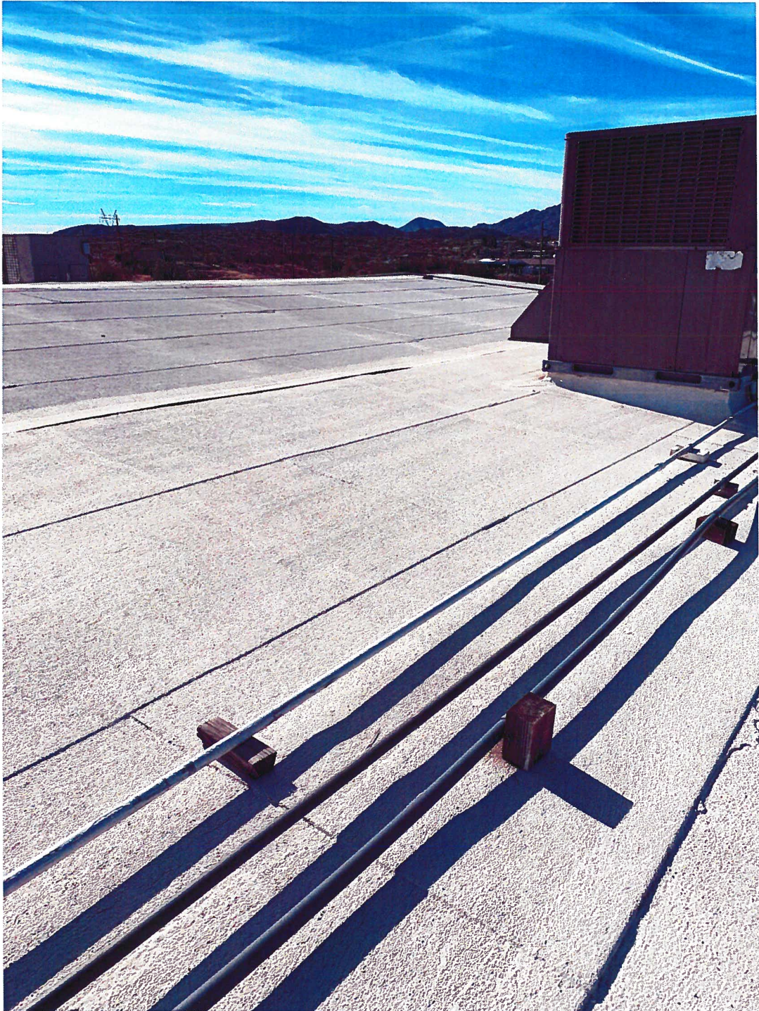
Building 1002 Typical Condition (Upper Roof)
